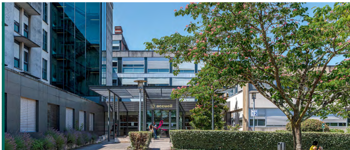
Pont de Chaume private hospital, Montauban (82) – Elsan
