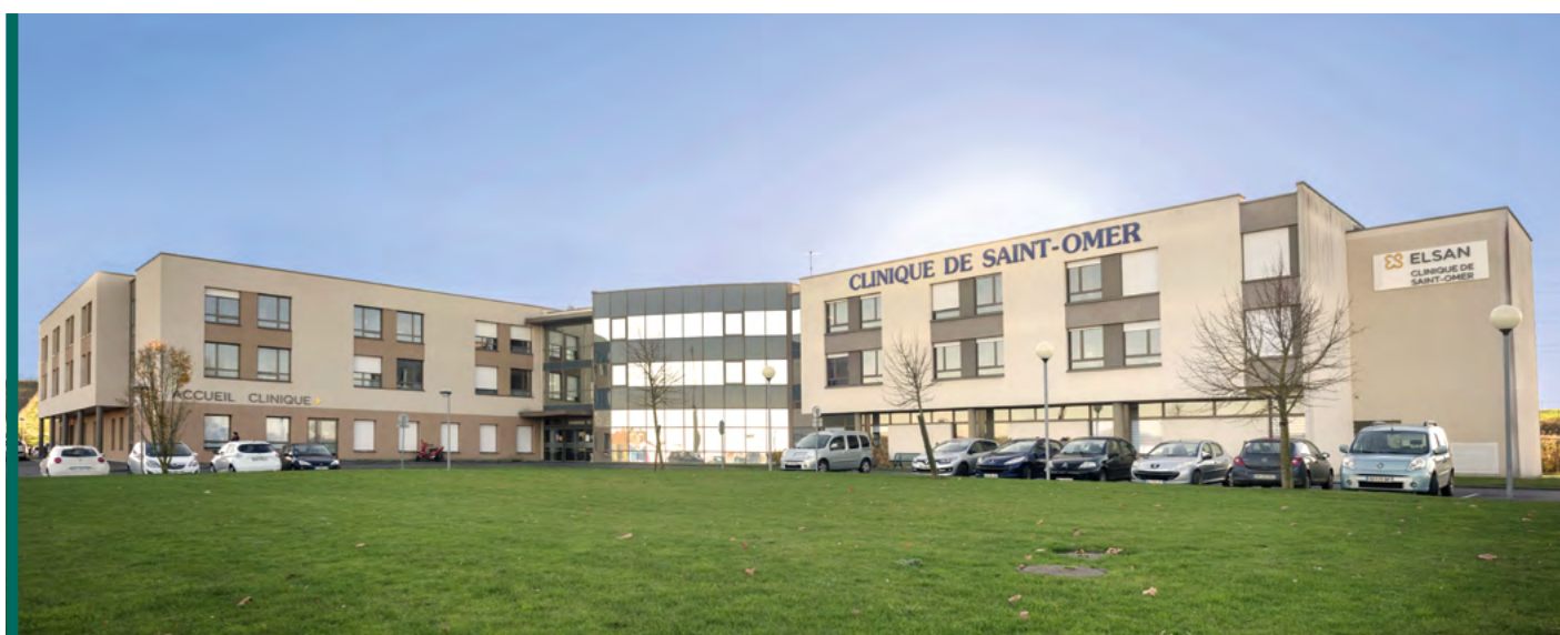
Saint-Omer private hospital, Blendecques (62) – Elsan
