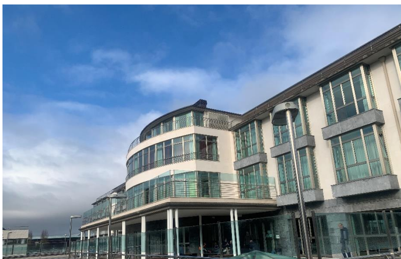
Long-term care facility, Spain
