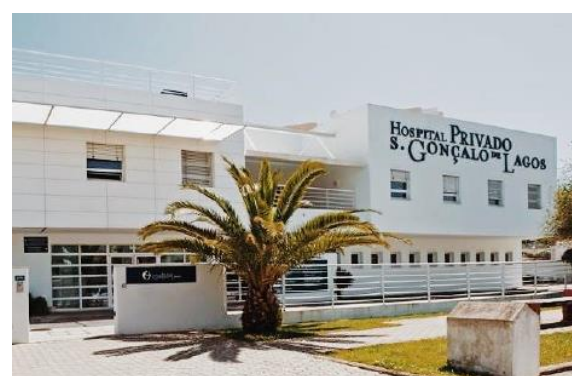
Hôpital de Lagos (HPA Saúde) – Algarve, Portugal
